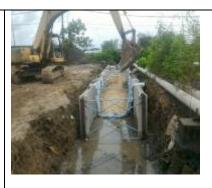
SPS System with panels, bracings, geotextile put together
