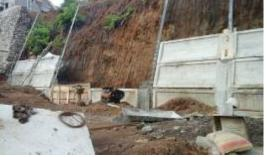
SPS System panels above the foundation panels (lowest panel sets) are leaning towards the slope
