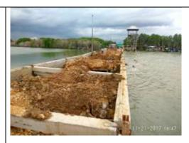
SPS Construction replaced the previous conventional wave breaker and also utilized as road
